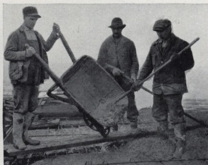
Pouring concrete for the roof. The entire roof should be placed in one continuous operation to secure a watertight job
