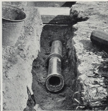
Pack joints of the sewer pipe with cement mortar. Best grade for inlet is \frac{1}{4} inch to the foot. Too steep a fall should be avoided
