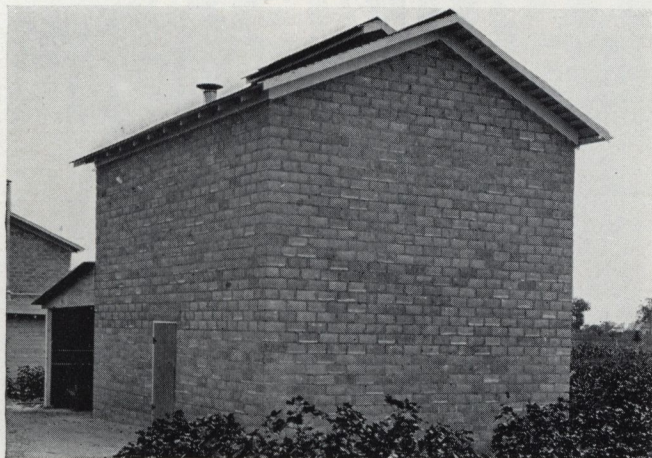
Tobacco Curing Barn built with concrete block. Excellent results have been obtained with this permanent and fireproof structure
