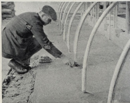
Mounding the concrete in a cone around the stall partitions prevents rusting of metal where it enters the concrete
