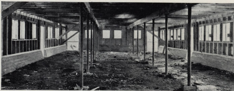
Interior of a dairy barn, ready for the placing of a concrete floor. Note the concrete foundation wall. Concrete foundations support the posts. A 1:2½:4 concrete mixture (1 part cement, 2½ parts sand, and 4 parts gravel or stone) is recommended for barn floors
