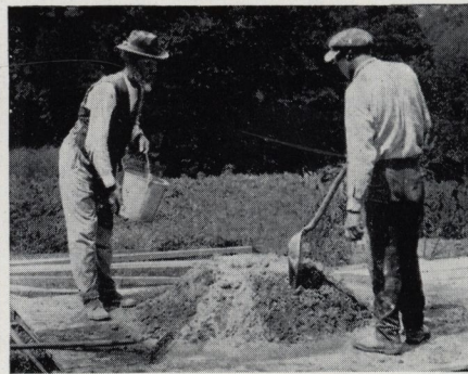
Make a hollow in the center of the pile and add water
