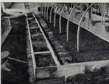
Floor and alley forms over the gutter foundation. A little soil placed in forms holds them in place while pouring the concrete
