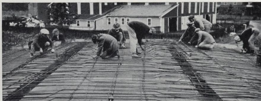
Placing the reinforcing for the roof. The roof should be built under the supervision of a contractor experienced in reinforced concrete slab construction. The reinforcing rods can be purchased ready to place in position. The manufacturer will furnish a plan
