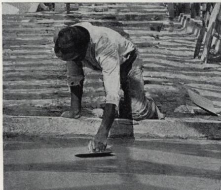
Poultry house floors should be given a smooth surface with a steel trowel. Rough finished floors wear away toe-nails of birds
