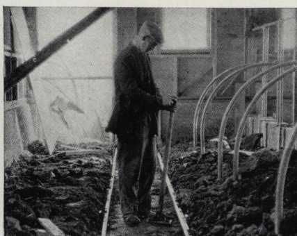
The earth foundation should be wet down and thoroughly tamped to insure solid packing before pouring concrete
