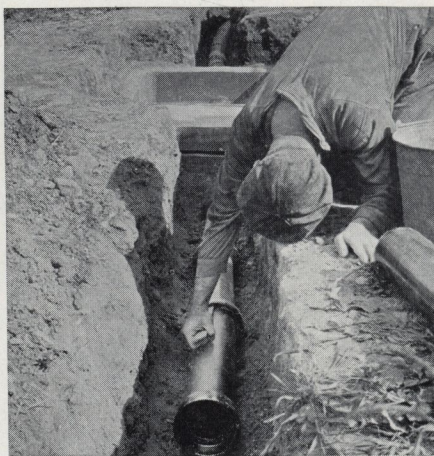
Force a few strands of oakum or shredded tarred rope in bell end of sewer pipe before cementing the joint
