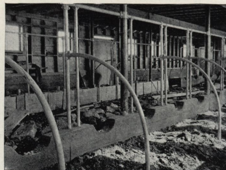
Curb with forms removed. A lower curb, with no cut-out, can be used if desired. Low level curb should be 6 inches high
