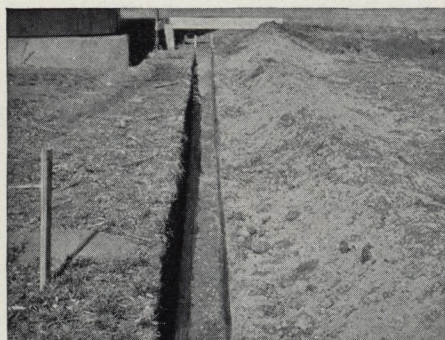
Trench for foundation wall. Where the soil is firm and has been carefully dug, forms are not necessary
