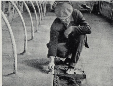
Finishing with an edger to produce a rounded corner, preventing the concrete from chipping. Avoid sharp corners
