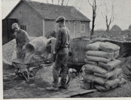
Turn the drum to the other side of the mixer and dump the thoroughly mixed concrete into a wheelbarrow
