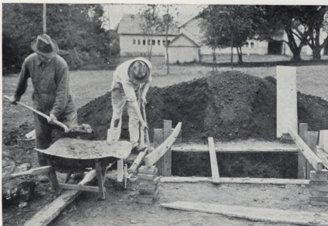
Placing the concrete. A 1:2:4 mix is recommended, made very stiff. Pour walls first, and then the floor, in one operation. Tamp concrete continually while pouring
