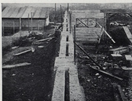
View along top of wall. Note the dead air space between outer and inner walls except at pilasters
