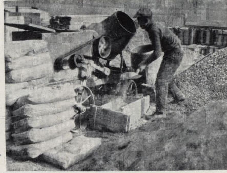
Add the cement. A box to hold the cement supply is advisable, as only a small amount is needed for each batch
