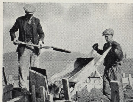
A few boards used to direct the concrete while pouring will prevent the loss of materials over side of forms
