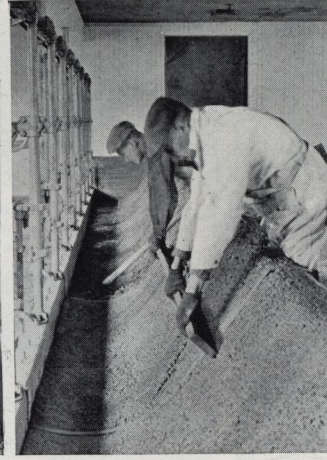
Striking off the concrete, using the metal templates as guides for the straightedge
