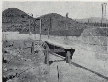
Wall partly completed. The dark layer of concrete at top of wall is a fresh course made with the double wall molds
