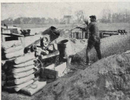
A concrete mixer operated by a gas engine saves much of the hard work in mixing, and makes better concrete
