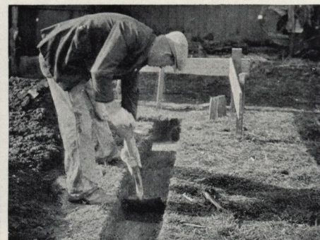
Tamp concrete into place to get a compact wall, with no air pockets that require patching when forms are removed
