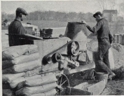
Allow the mixing to continue for at least a minute. Longer mixing will give stronger concrete
