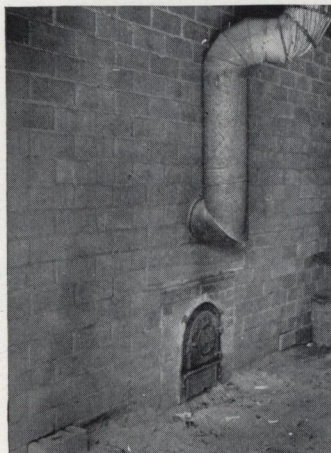
Furnace and flue. Note removable blocks in bottom course, for ventilation
