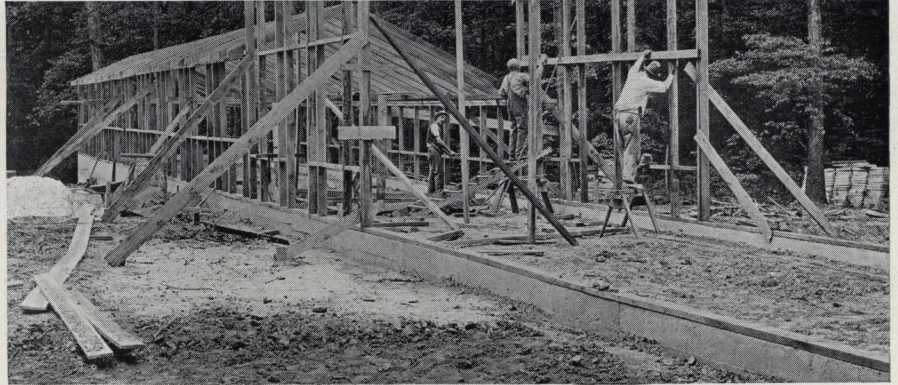
Ready for the concrete floor. A mixture of 1:2:3½ concrete (1 part cement, 2 parts sand, and 3½ parts gravel or stone) is recommended for both foundation wall and floor. Gravel or stone up to one inch in size can be used in mixing the concrete
