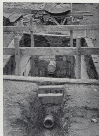
The concrete must be packed thoroughly under and around the Y-branches
