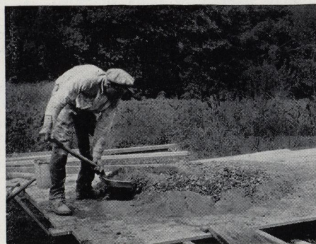
Add desired quantity of pebbles or broken stone, and mix thoroughly
