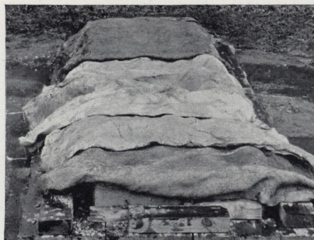
Cover the entire form with straw or burlap, and keep wet by sprinkling until the posts are removed from forms
