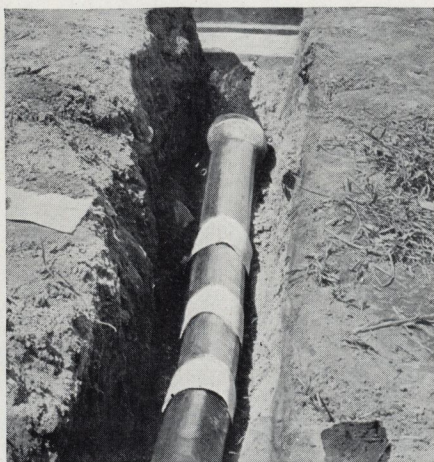
Farm drain tile, 3 or 4 inches inside diameter, one foot long, is used for outlet. Place tar paper over joints to keep soil out
