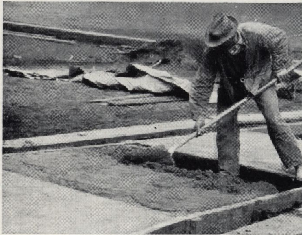
Use water sparingly in mixing concrete. Within reasonable limits, the less water used, the better the concrete
