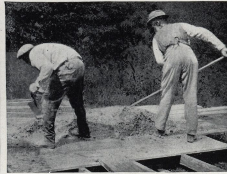
Mix until desired consistency is obtained, adding more water if necessary
