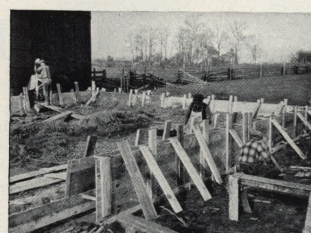
Forms for the wall are built over the foundation. Bolts to fasten the sill are placed in position in the forms
