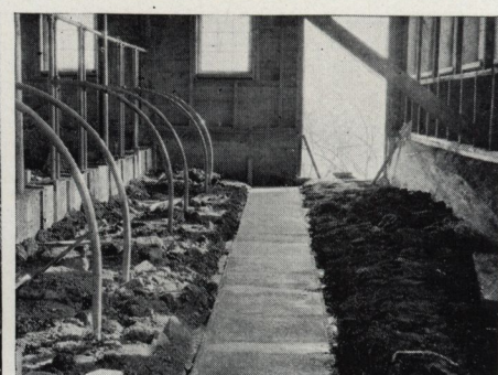
The bottom of the concrete gutter should be wide enough to allow stall and alley floors to overlap several inches
