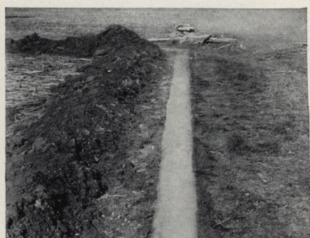
Foundation for the wall poured to the ground level. The section of the wall above ground can now be constructed
