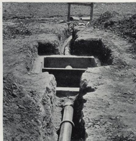
The completed tank (without cover slabs), showing inlet line of sewer pipe and the outlet line of drain tile in place
