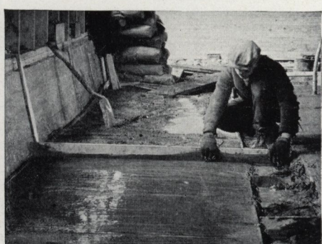
Leveling the concrete in the litter alley. For good drainage, the incline from foundation wall to gutter should be one inch
