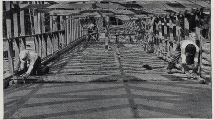
Leveling the concrete. Note how the 2 x 4's at the sides furnish a guide for the strike-off board. Expansion joints of several layers of roofing paper should be placed between wall and floor
