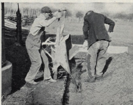
Placing the concrete. A mix of 1 part cement, 2\frac{1}{2} parts sand and 4 parts gravel or stone is recommended for foundations
