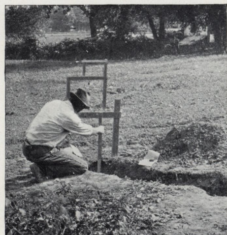
Drainage line should have a fall of 2 inches in 100 feet. Use at least 100 feet of tile. More will be needed in poorly drained soil
