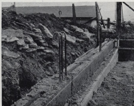
Footing and first course of wall completed. Note the reinforcing rods placed in the concrete for the pilaster
