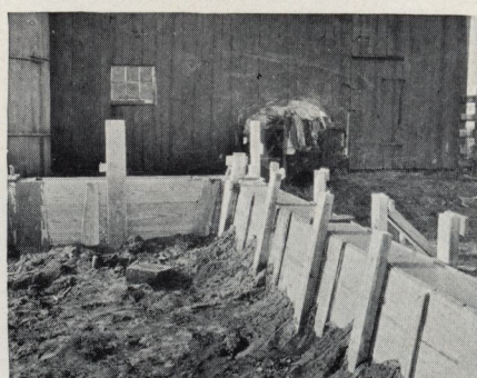
Wall forms completely filled. Concrete should be spaded while it is being poured, to secure a surface free from air holes
