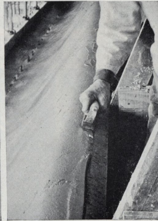
A rounded edge improves the appearance and prevents corners from chipping
