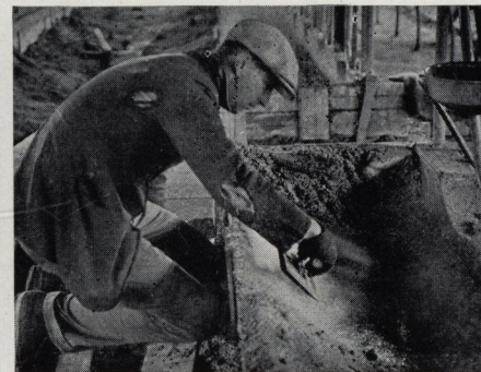
A steel trowel produces a smooth, easily cleaned surface. Do not use trowel more than necessary to obtain smoothness
